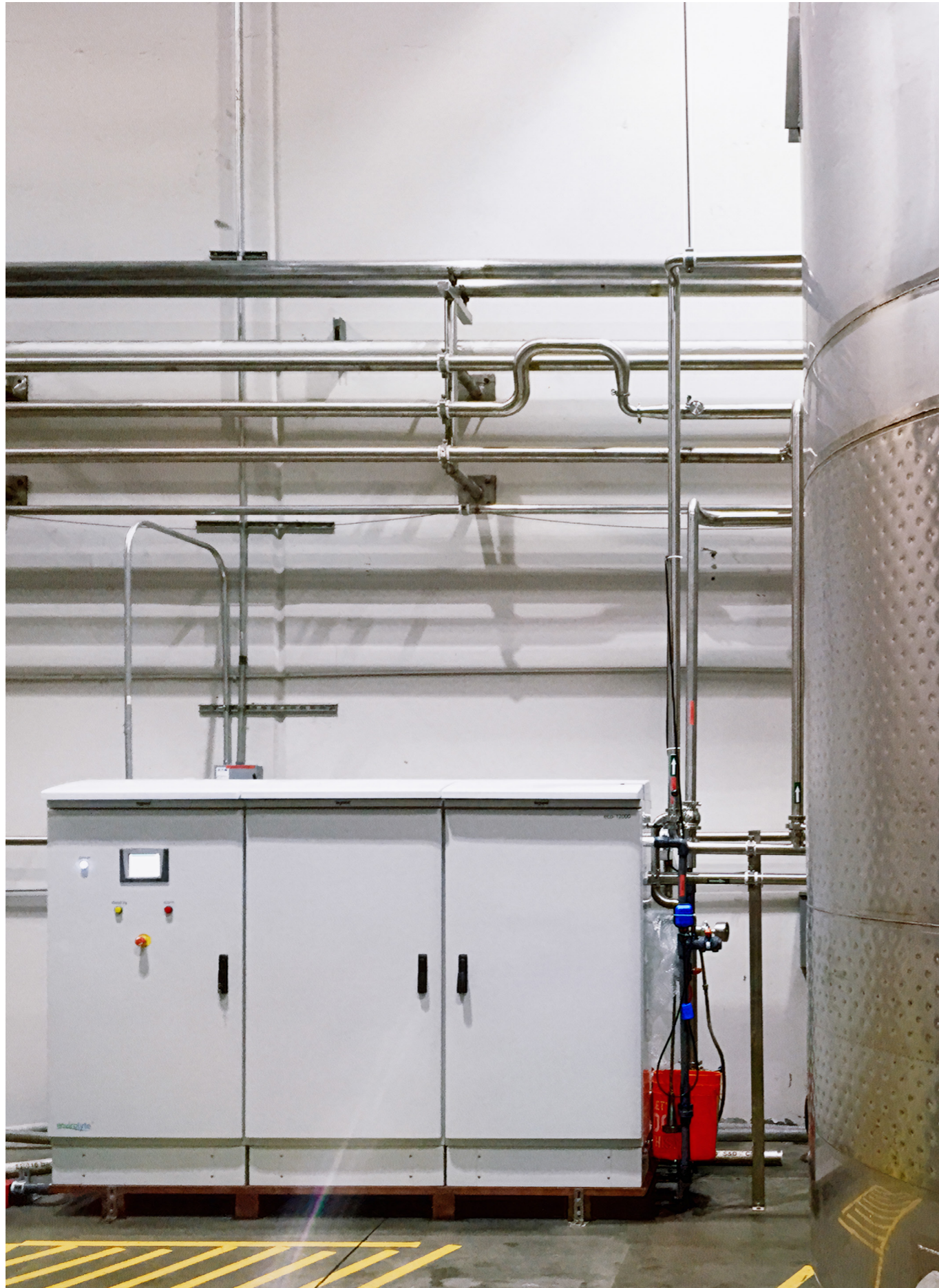
Enviolyte eco12000 alkaline ionized water generator at a bottling plant in USA
